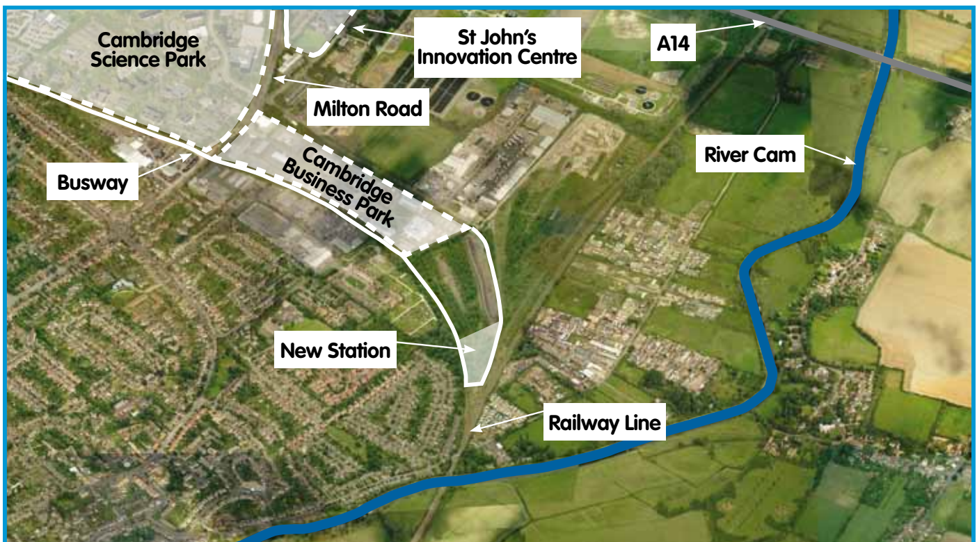
Aerial view of the site of the new station and surrounding areas
